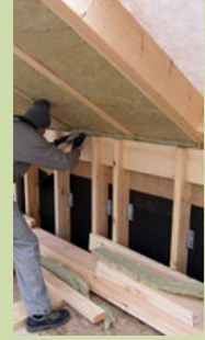
Roof insulation
