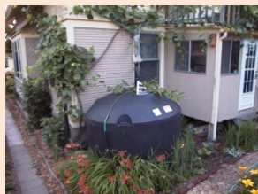
Rainwater harvesting system
