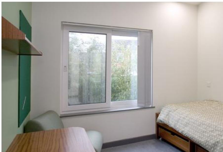
Figure 18 Example of a suitable secure window with mesh for a mental health patient bedroom
