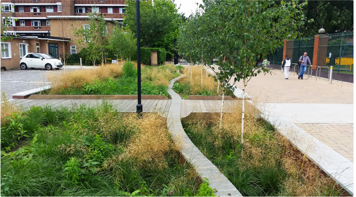
A sustainable urban drainage system at work - 'there is potential benefit in exploring the introduction of a sustainable drainage offset policy'
